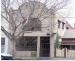
fitzroy north nicholson street fitzroy north nicholson street 424
