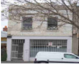
fitzroy north nicholson street fitzroy north nicholson street 426
