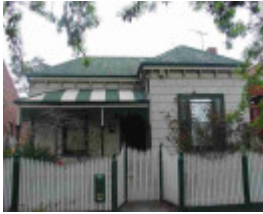
fitzroy north rushall crescent fitzroy north rushall crescent 11
