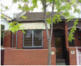
fitzroy north holden street fitzroy north holden street 57
