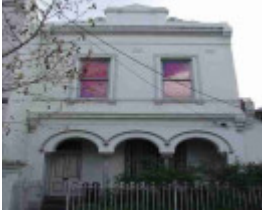
fitzroy kerr street fitzroy kerr street 31
