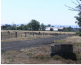
DEANSIDE WOOLSHED COMPLEX SOHE 2008
