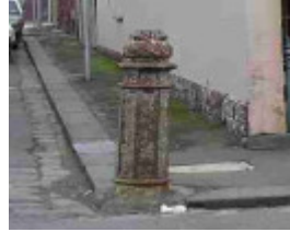
Cast Iron Pillar.JPG
