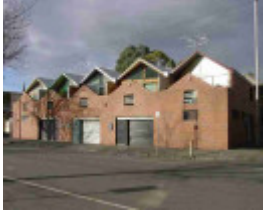
fitzroy napier street fitzroy napier street 144-152, part
