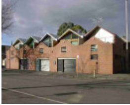
fitzroy napier street fitzroy napier street 144-152, part
