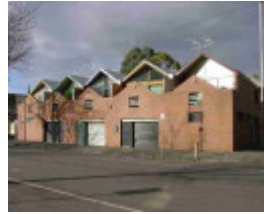
fitzroy napier street fitzroy napier street 144-152, part
