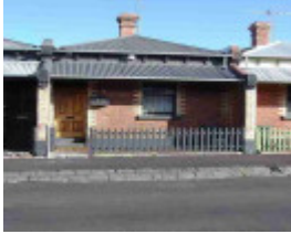
fitzroy garfield street fitzroy garfield street 10
