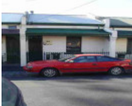
fitzroy garfield street fitzroy garfield street 11
