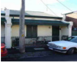
fitzroy garfield street fitzroy garfield street 13
