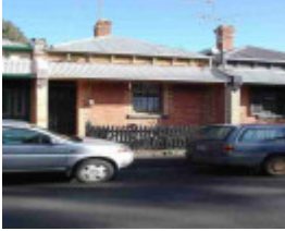
fitzroy garfield street fitzroy garfield street 14
