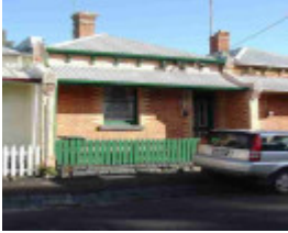
fitzroy garfield street fitzroy garfield street 16
