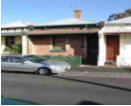
fitzroy garfield street fitzroy garfield street 20
