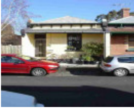
fitzroy garfield street fitzroy garfield street 22
