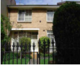
fitzroy hanover street fitzroy hanover street 34
