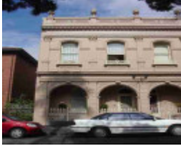
fitzroy hanover street fitzroy hanover street 38
