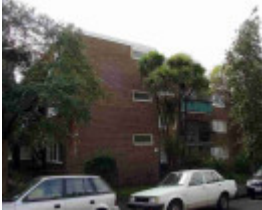
fitzroy hanover street fitzroy hanover street 41
