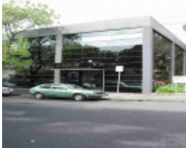
Fitzroy Hanover Street 60-66.JPG
