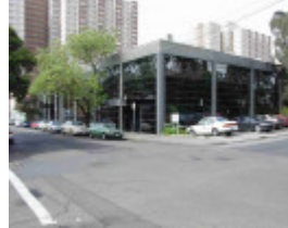
Fitzroy Hanover Street 60-70.JPG
