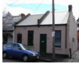
Fitzroy Hanover Street 69- 71.JPG
