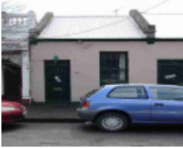
fitzroy hanover street fitzroy hanover street 69
