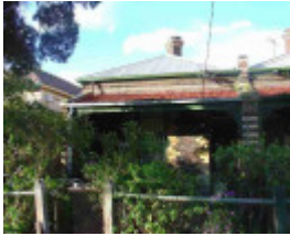
fitzroy north michael street fitzroy north michael street 80
