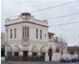
fitzroy north nicholson street fitzroy north nicholson street 414
