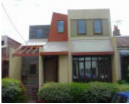
fitzroy north liverpool street fitzroy north liverpool street 5
