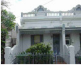
fitzroy north liverpool street fitzroy north liverpool street 9
