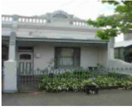
fitzroy north liverpool street fitzroy north liverpool street 11
