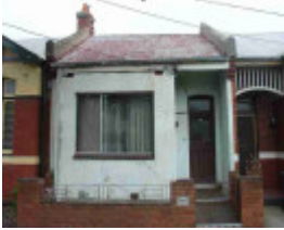
fitzroy north holden street fitzroy north holden street 53
