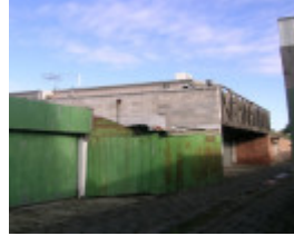
Rear of 91 Clauscen Street.JPG
