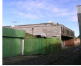
Rear of 91 Clauscen Street.JPG
