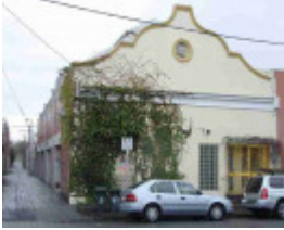
fitzroy westgarth street fitzroy westgarth street 93 unit 3
