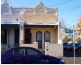
fitzroy north grant street fitzroy north grant street 14
