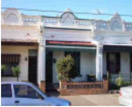
fitzroy north grant street fitzroy north grant street 18
