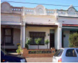
fitzroy north grant street fitzroy north grant street 20
