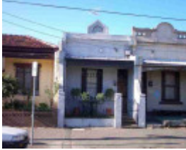
fitzroy north grant street fitzroy north grant street 24
