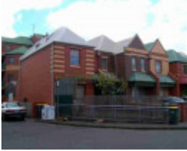
fitzroy north holden court fitzroy north holden court 3
