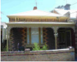
fitzroy north ivan street fitzroy north ivan street 21
