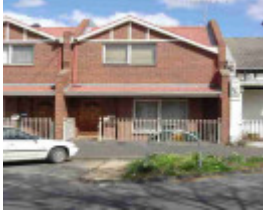
fitzroy westgarth street fitzroy westgarth street 16 unit 1
