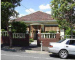
richmond docker street richmond docker street 53
