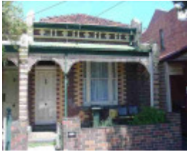
fitzroy north church street fitzroy north church street 40
