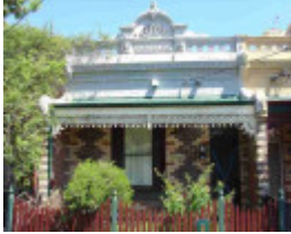
fitzroy north bennett street fitzroy north bennett street 23
