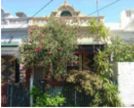
fitzroy north bennett street fitzroy north bennett street 25
