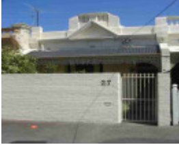
fitzroy north bennett street fitzroy north bennett street 27
