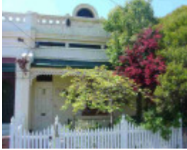
fitzroy north bennett street fitzroy north bennett street 28
