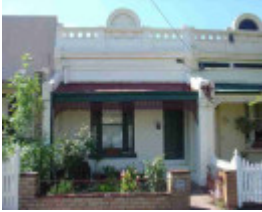
fitzroy north bennett street fitzroy north bennett street 30
