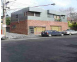
fitzroy hanover street fitzroy hanover street 14
