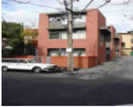
fitzroy hanover street fitzroy hanover street 18 unit 1-3
