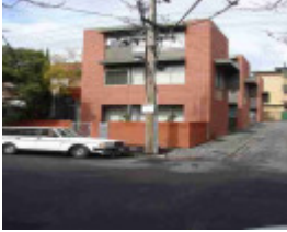
fitzroy hanover street fitzroy hanover street 18 unit 1-3
