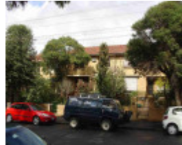
Fitzroy Hanover Street 20- 26.JPG
