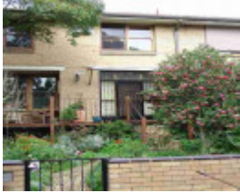
fitzroy hanover street fitzroy hanover street 22
