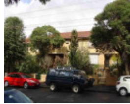
Fitzroy Hanover Street 20- 26.JPG
