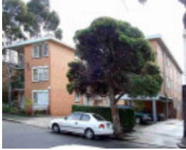
fitzroy hanover street fitzroy hanover street 27
