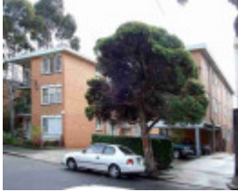
fitzroy hanover street fitzroy hanover street 27
