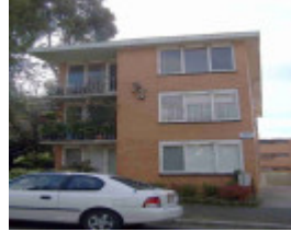
Fitzroy Hanover Street 027.JPG
