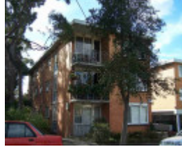
Fitzroy Hanover Street 027.JPG
