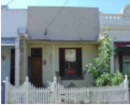
fitzroy north bennett street fitzroy north bennett street 32
